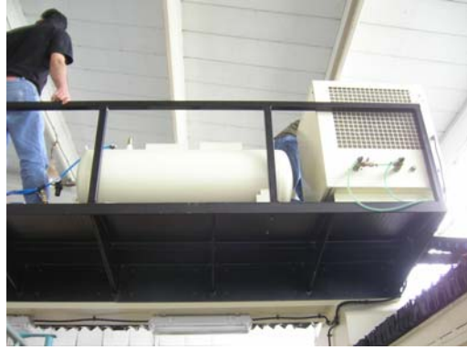
ON THE BRIDGE INSTALLED COOLING UNIT
